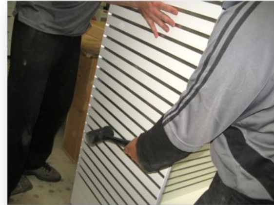
9. using soft hammer gently knock end panel into place until flush with
